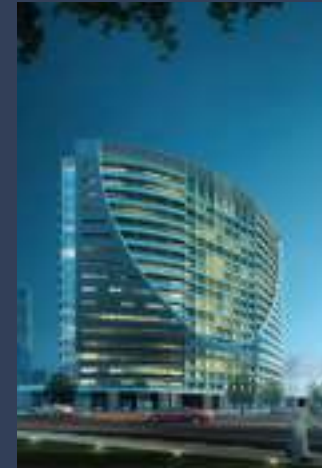
The V Tower
